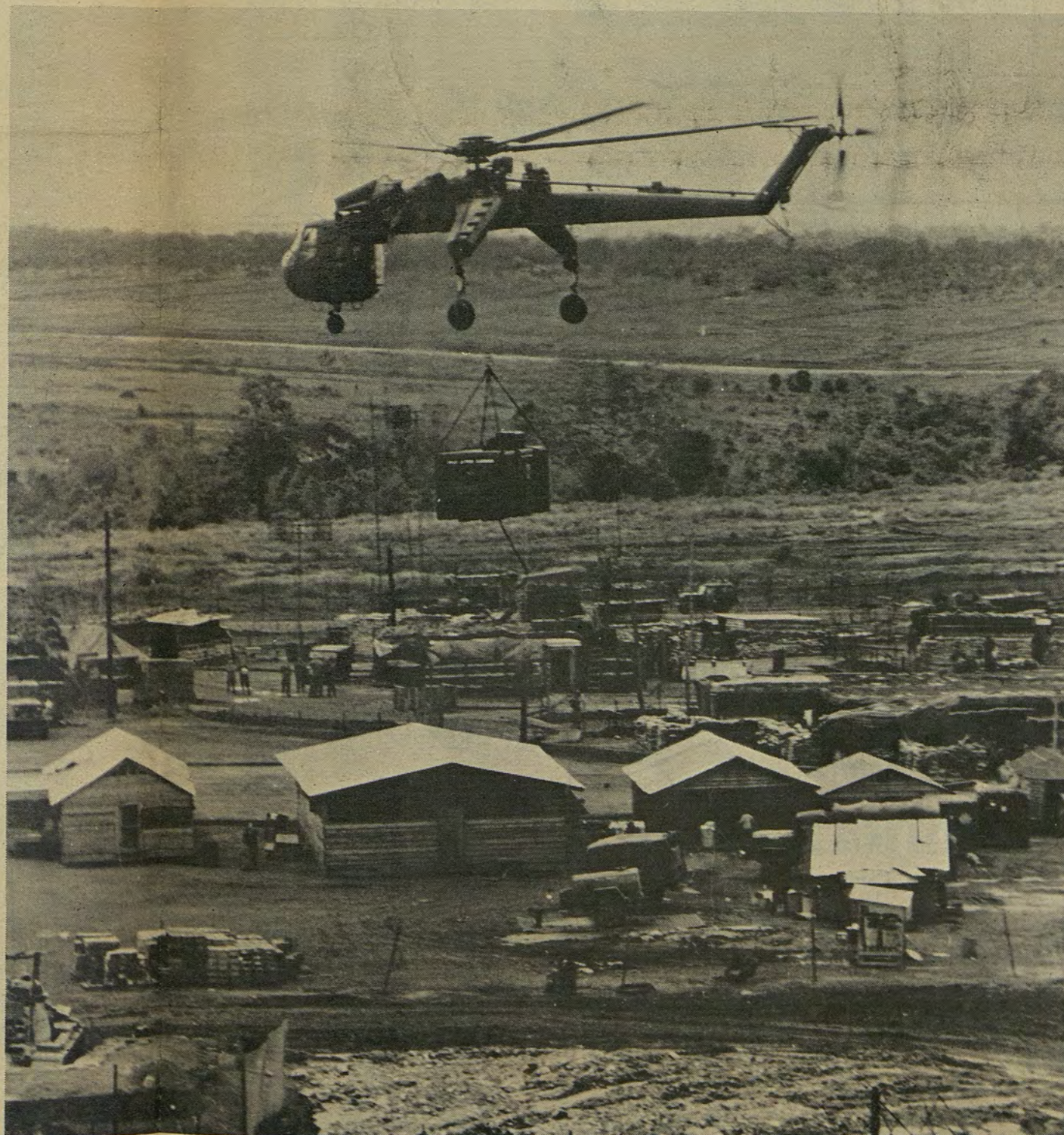
A HUGE "FLYING CRANE" HELICOPTER DEPOSITS CLINIC AT BLACKHAWK FIREBASE. USA Photo by PFC Gordon May
